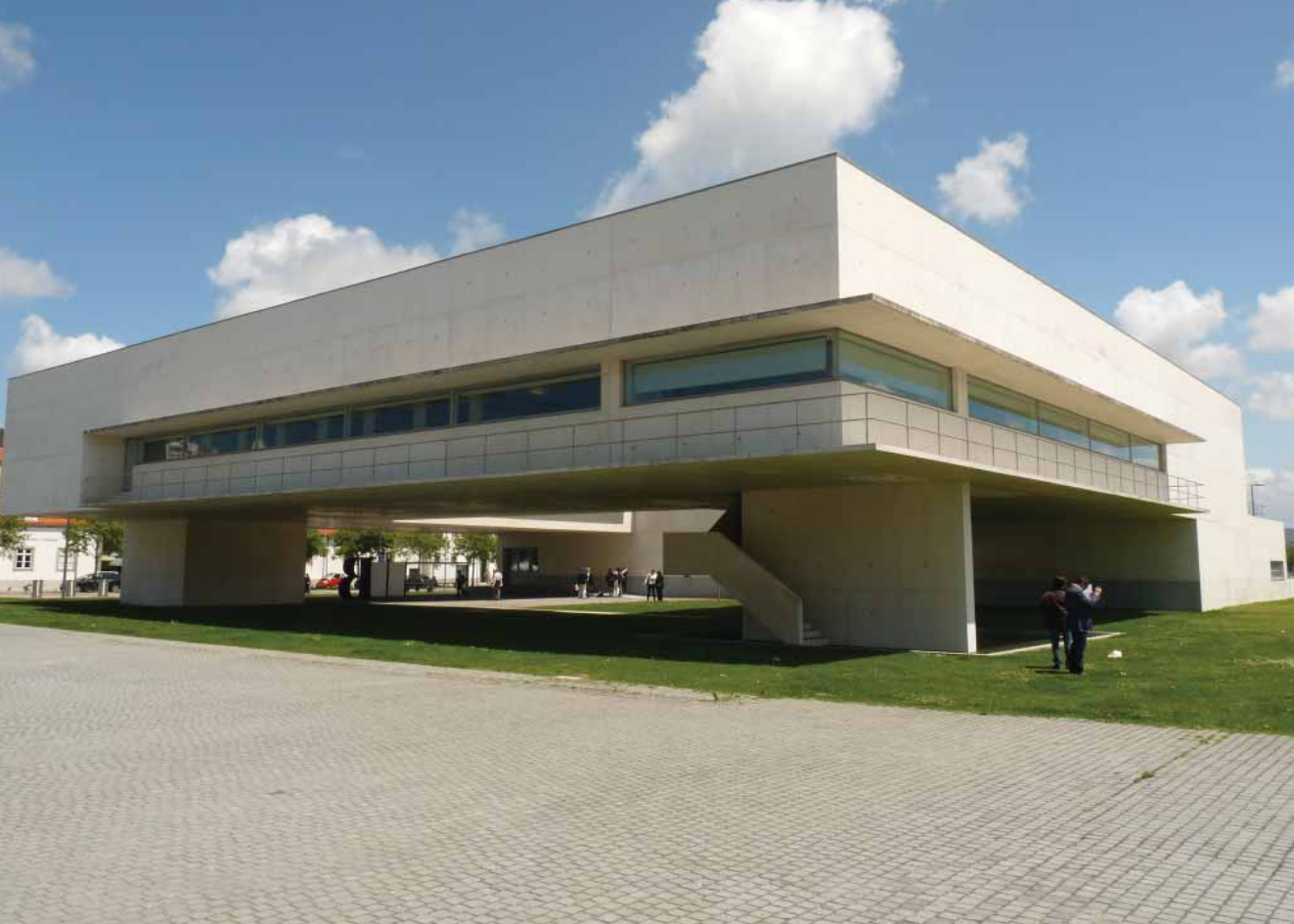
Fig. 08: New strategic equipments on the river bank. (© Ana Félix, Fernando Flores, Alberto Monteiro)
