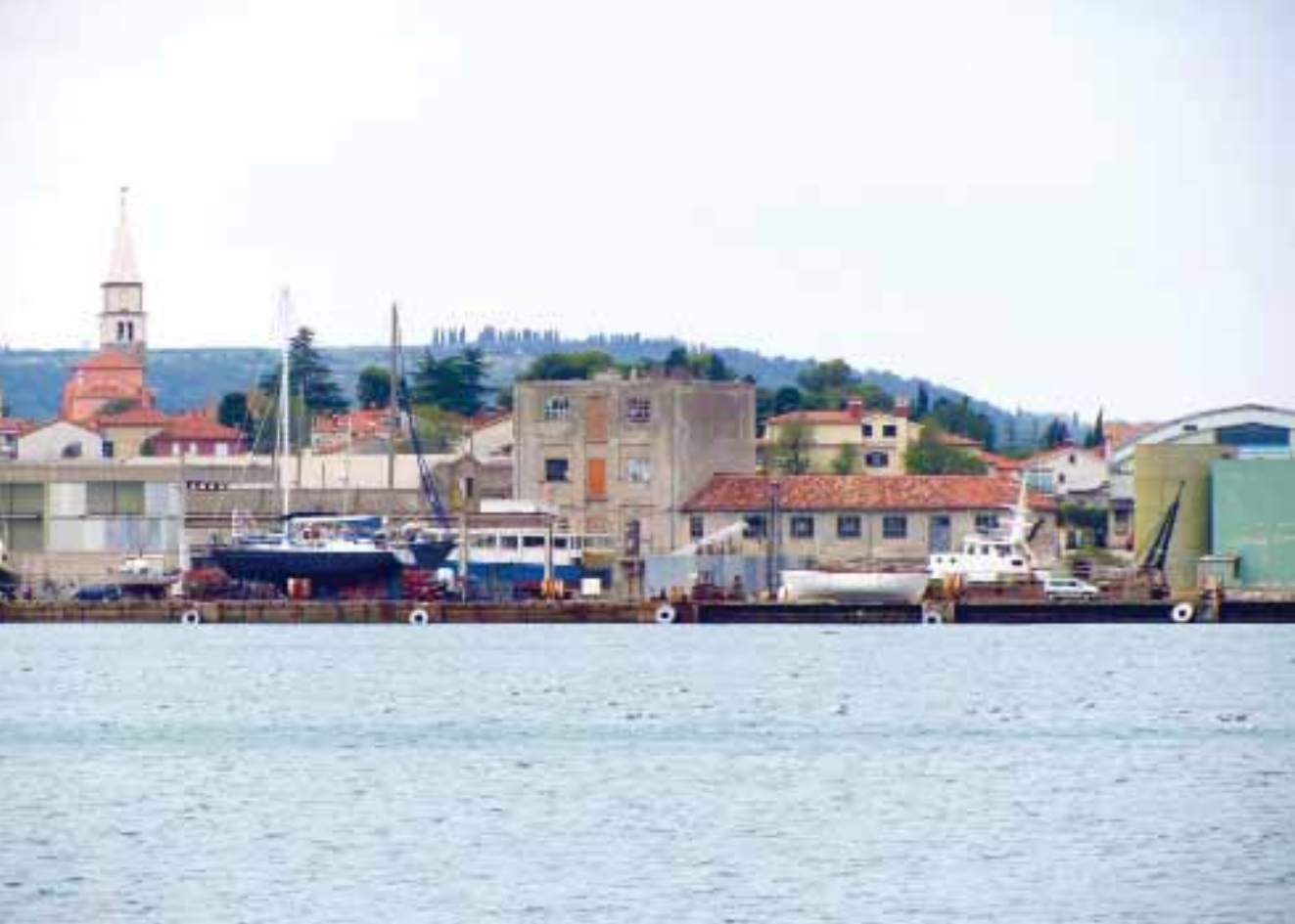
Fig. 04: Brownfield area (abandoned Izola shipyard) due to lack of effective spatial planning. (© Tadej Podakar)
